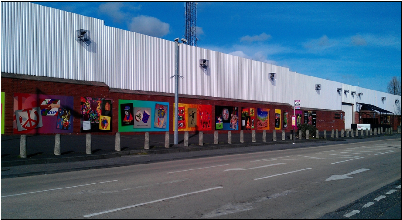
Murals created by young people as part of the SLIG sponsored Woodbourne improvement scheme add a bright a cheerful note to the heavily fortified Woodbourne police station.
