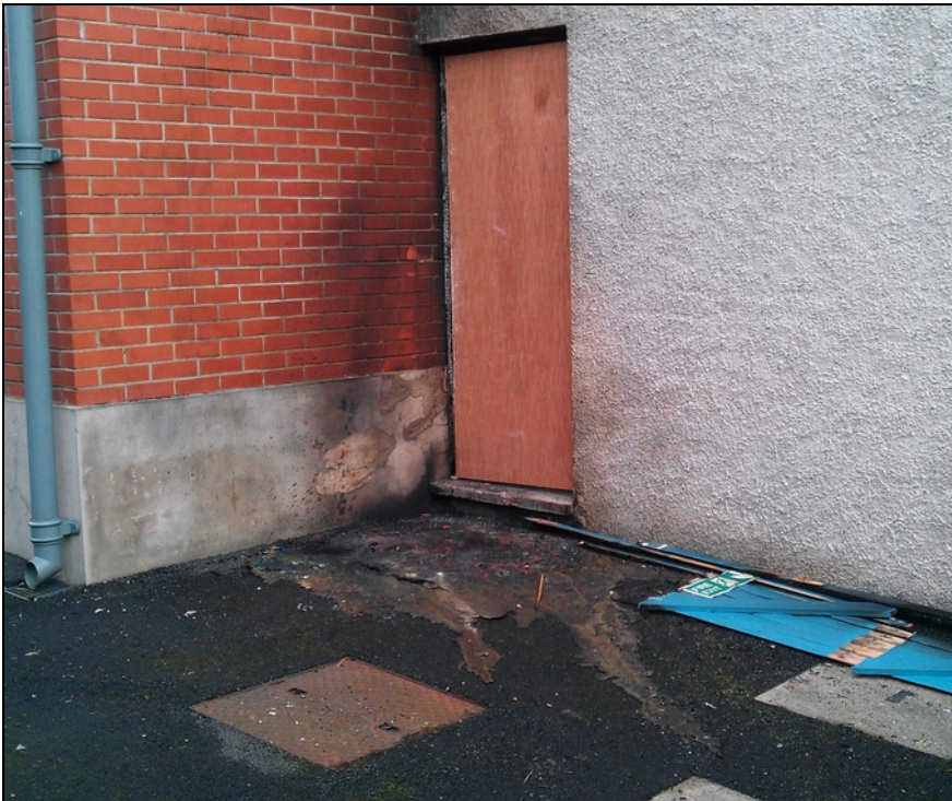
Fire damage to wooden door, wall render, and bitmac surface. Stolen bread trays had been placed against the door and ignited.
