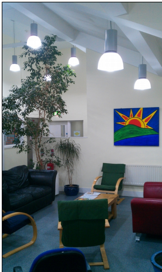
Daylight colour 23 watt LED lamps replace 58 watt fluorescent fittings in the lobby
